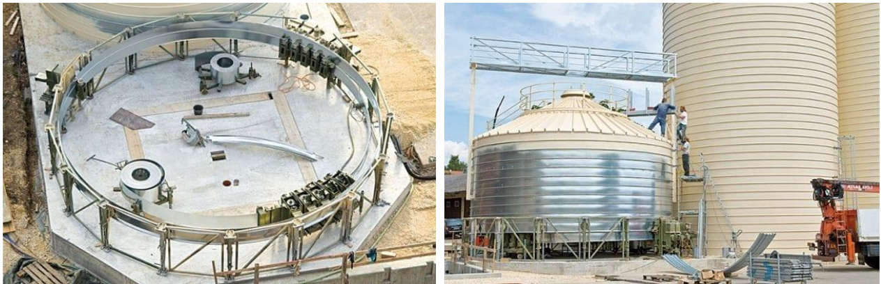
Fig.2. Stages of assembling a spiral-fold silo [https://xaver-lipp.com/]
