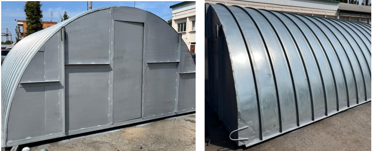
Fig. 8. The completed structure
