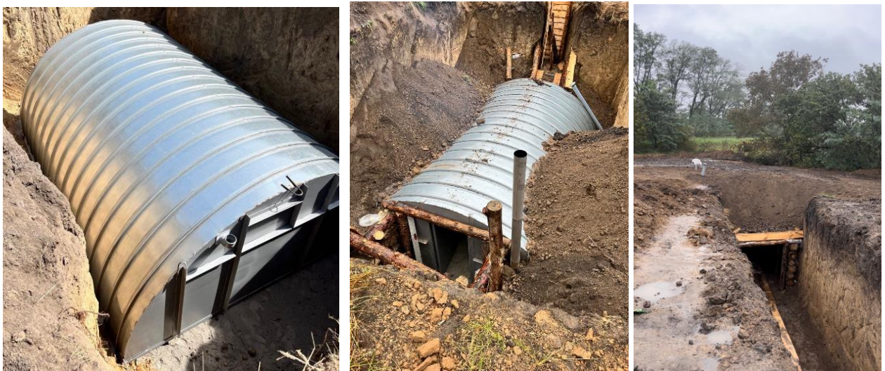
Fig. 9. Installation of the shelter
