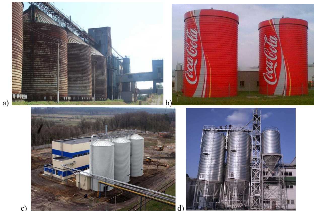
Fig. 3. Spiral-fold structures are applied in various industries in Ukraine: a) grain silos; b) water tanks [ https://www.lipp-system.de/tanks/?lang=en ]; c) silos as storage for biomass[ https://watzenrode.com/ ]; d) sunflower husk silos;
